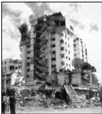
Fig. 3.3a: Destruction caused by an Earthquake at Bhuj
