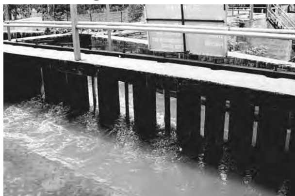
Fig. 18.4 Grit and sand removal tank
